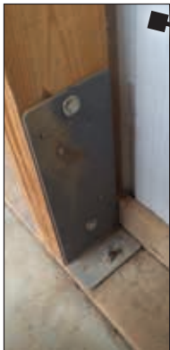
3- or 4-ply laminated column on concrete or in ground and have a 50-year warranty.
