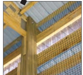
EPS truss to column connections are center mounted and bolted for superior strength.
