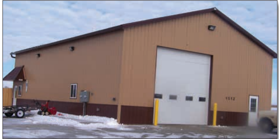
Welding shop, Sioux Falls, SD, 40 x 60 x 16 Heat source: In-floor heat and electric boiler
